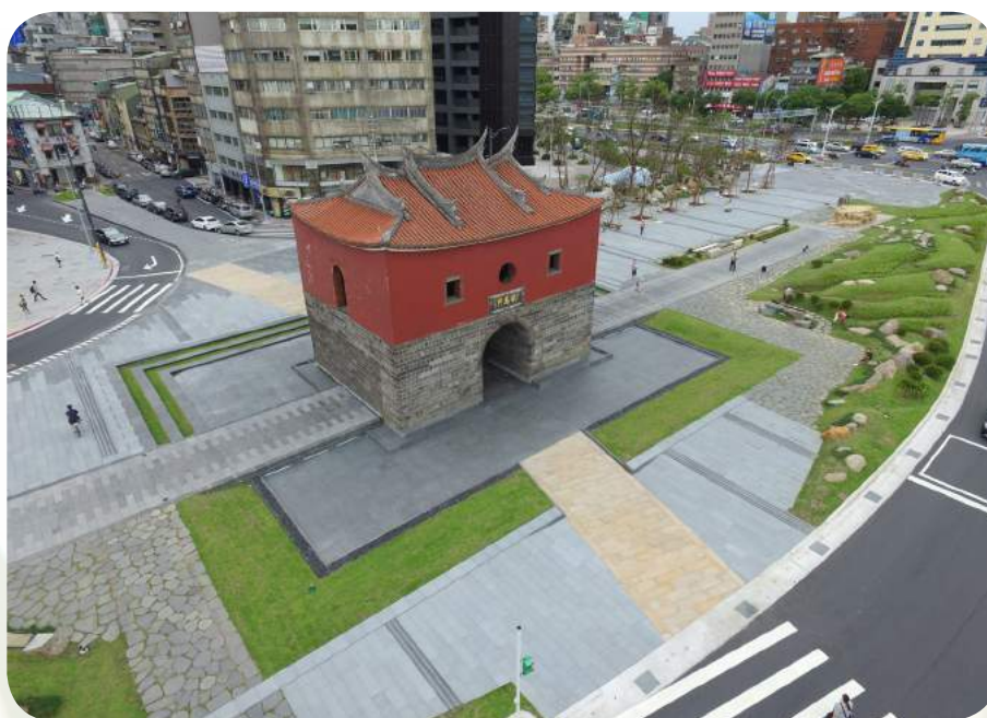
▲ Permeable pavement at the North Gate Square
