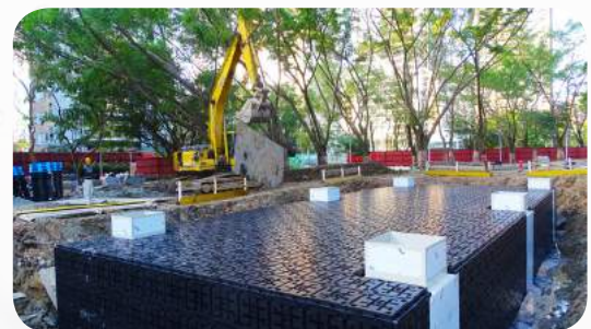
▲ Rainwater harvesting at Xiangshan Park
